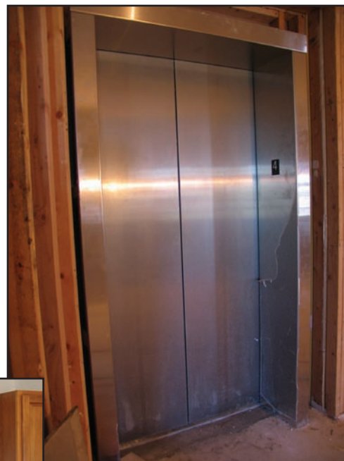
That 4th floor elevator now has a new stainless steel door.
