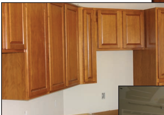
Cabinetry going into a 4th floor home.
