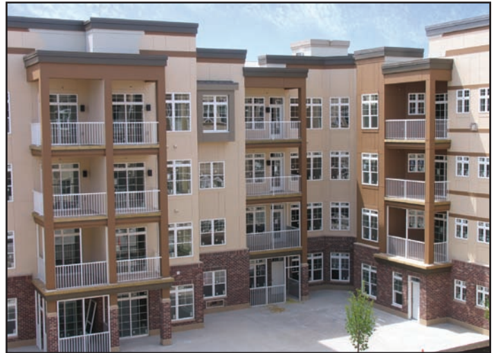
The Village Condominiums, Building Two
